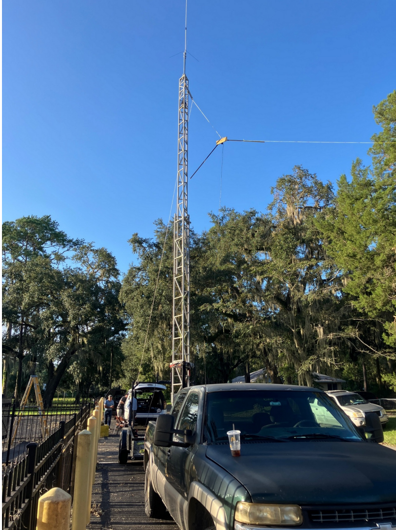
Figure 2: The completed antenna installation including vertical 2-meter antenna and homemade inverted V 6-meter antenna suspended by rope.
