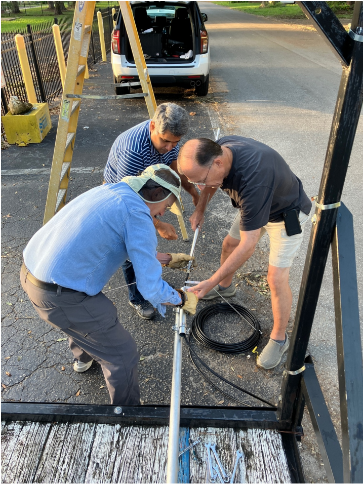
Figure 1: Attaching the 2-meter vertical antenna to the top of the mast.
