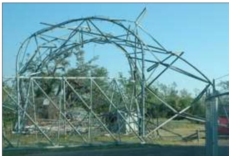
A downed communications tower, Plaquemines Parish, LA.
