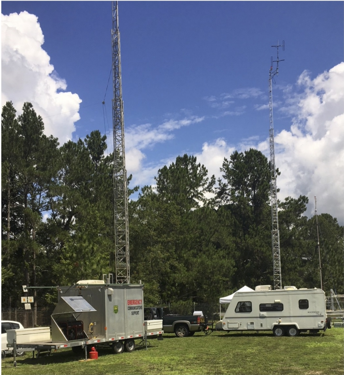
Two 100-foot towers and a refurbished travel trailer with a fiberglass mast. All with air conditioning.
